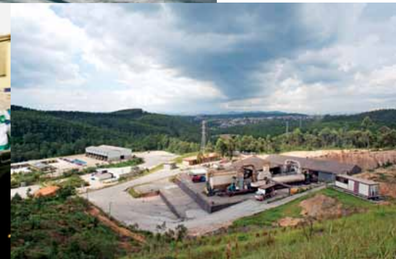
Essencis thermal desorption equipment at the Caieiras landfill (SP)
