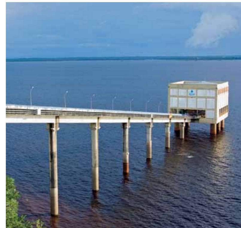
Water withdrawal lift station on the Rio Negro (AM)
