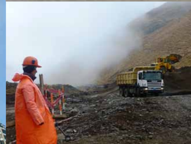
Vega Peru employees working on Andahuaylas / Kishuara highway
